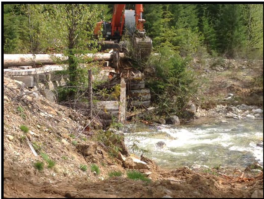
CK-2473 – Exposing Stringer Ends, Pulling Lashing
