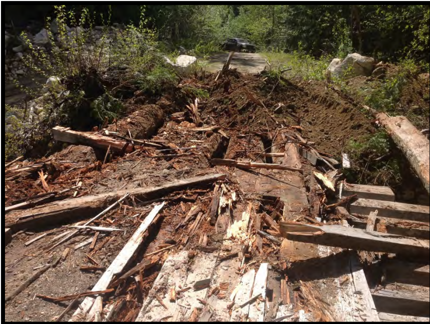
CK-2478 – Woods End Stringers Exposed
