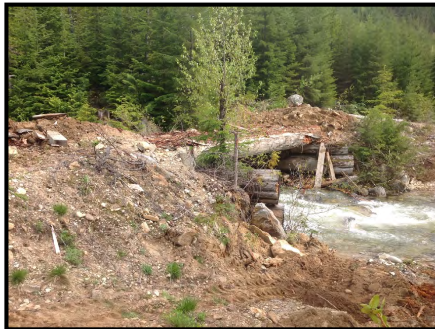
CK-2473 – All Deck Components Removed
