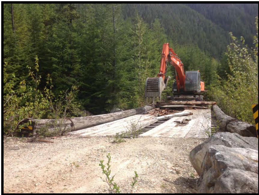
CK-2473 – Decking and Cross Tie Removal
