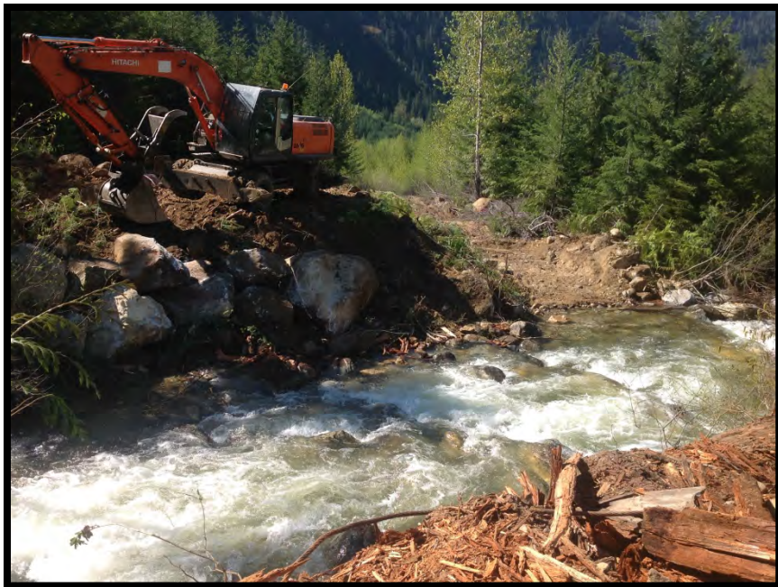
CK-2473 – Armoring Woods End Approach
