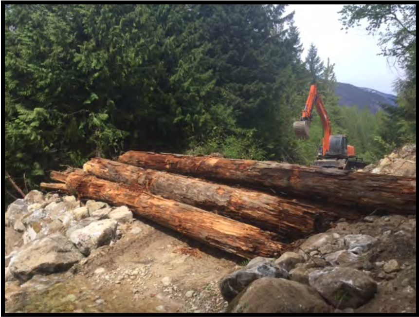
CK-2478 – Town End Approach Barricade, View from Channel
