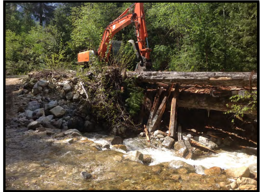
CK-2478 – Deck and Cross Tie Removal
