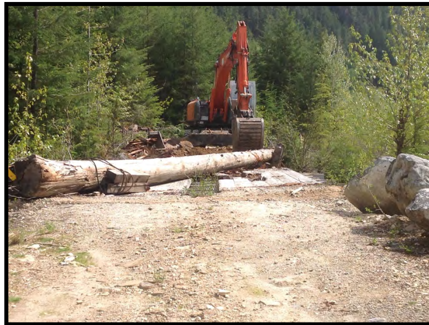
CK-2473 – Guard Log Removal
